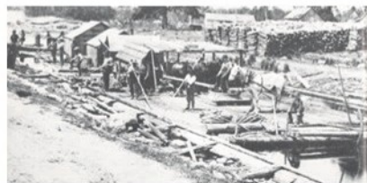
Raft of quality timber coming through the Bobcaygeon lock.
