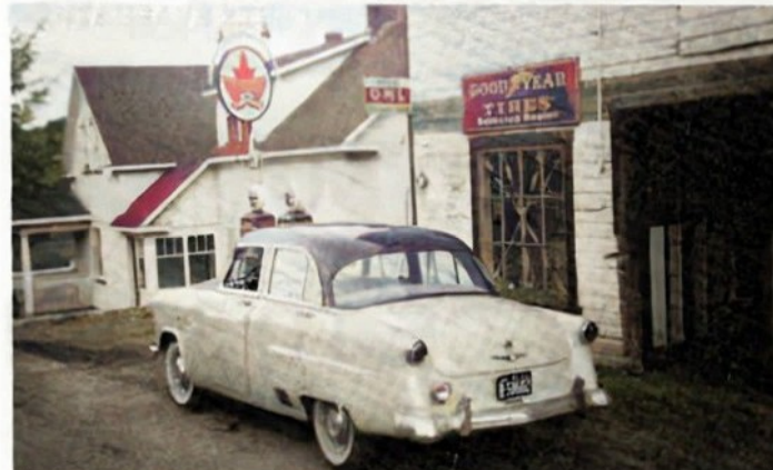
Supertest Gas pumps were installed at Simpson's Garage.
